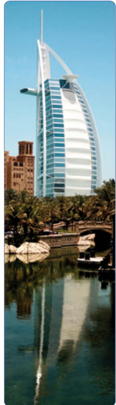
Burj Al Arab Hotel, Dubai, United Arab Emirates.
